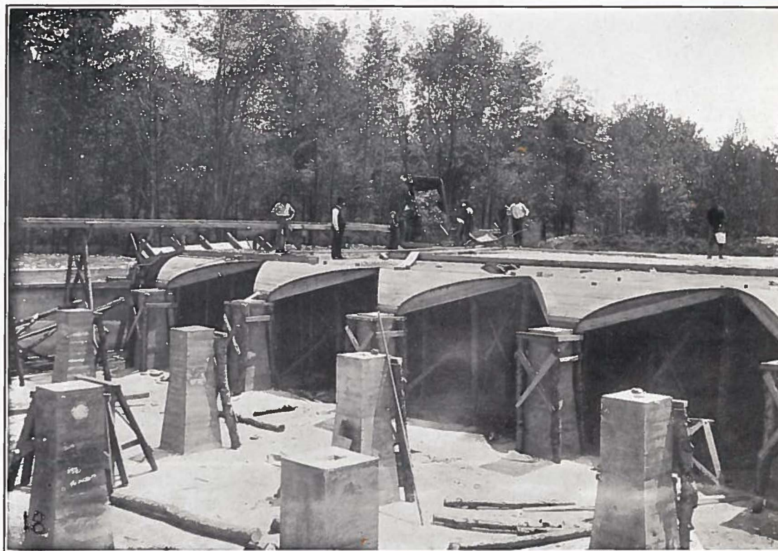
FIG. 8. SHOWING PIERS. CENTERING FOR ROOF. NO. 18
