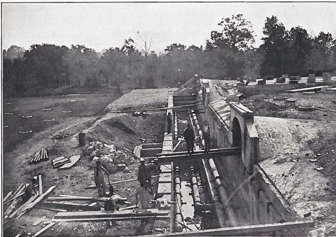
FIG. 7. PIPE GALLERY. BETWEEN PRIMARY AND SECONDARY FILTER. No. 38
