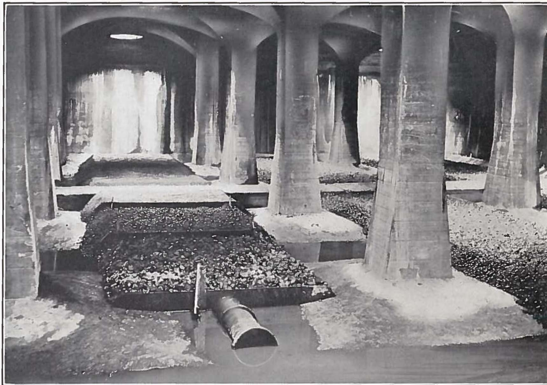
FIG 4. PRIMARY FILTER SECTION. LOOKING CROSSWISE. NO. 44
