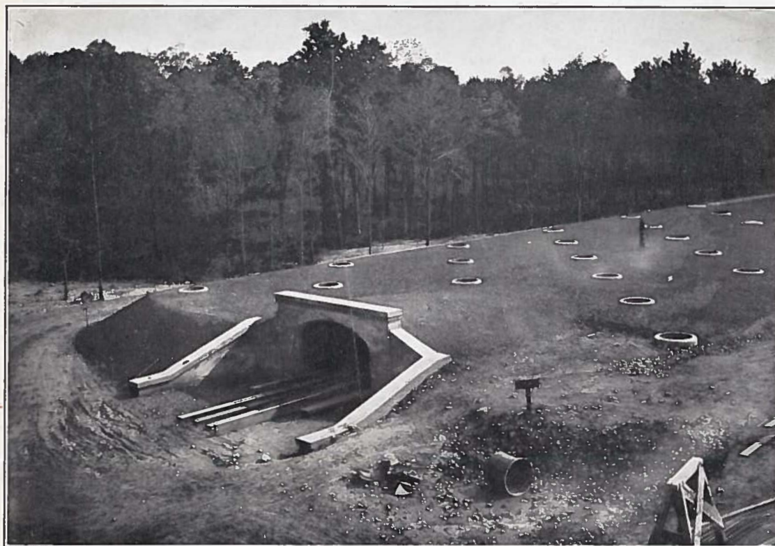
FIG. 3. SECONDARY FILTER. SHOWING ENTRANCE AND MANHOLES. No. 39
