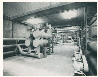
Fig. 1. Plant basement where chilled-water pumps, hot-water pumps, air compressors, and ventilation system are located. (Ed Stewart & Assoc. photo, Houston)
