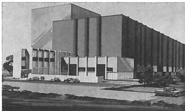
Offices are in foreground, turbine-generator room next and, just visible at rear is a building for housing a reactor.
