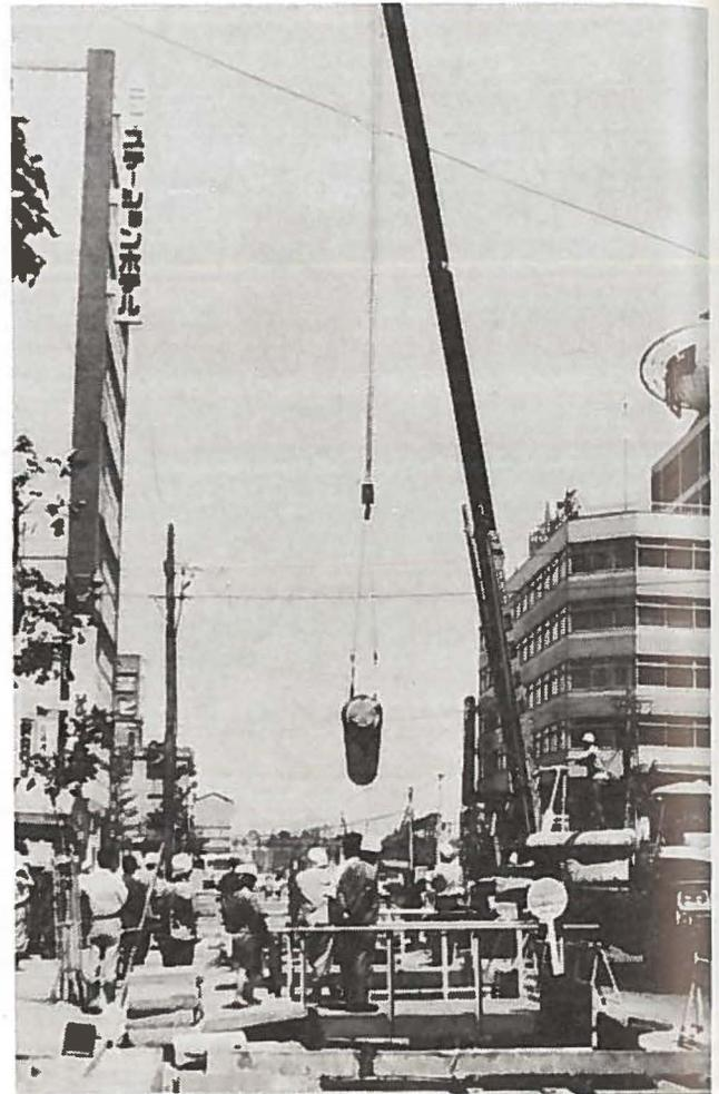
FIG. 2 — View of initial laying of conduit.
