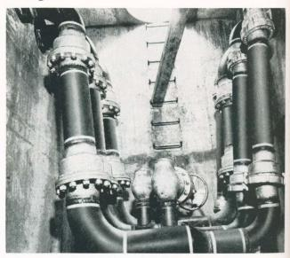
FIG. 3 — Ball joint installation in the high-temperature water system manholes.
