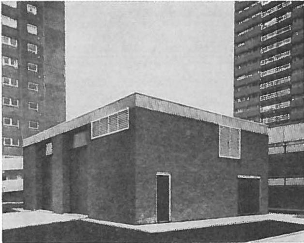
District heating without a single chimney: part of a gas-fired installation at Enfield (Photo by courtesy of the Eastern Gas Board)
