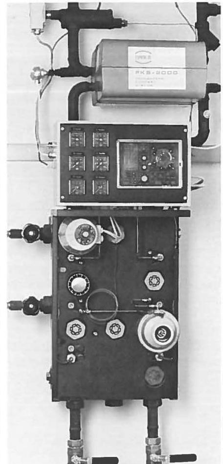
*Compact district heating transfer substations save both space and money. They can be fitted with all necessary devices required for heat transfer.*
