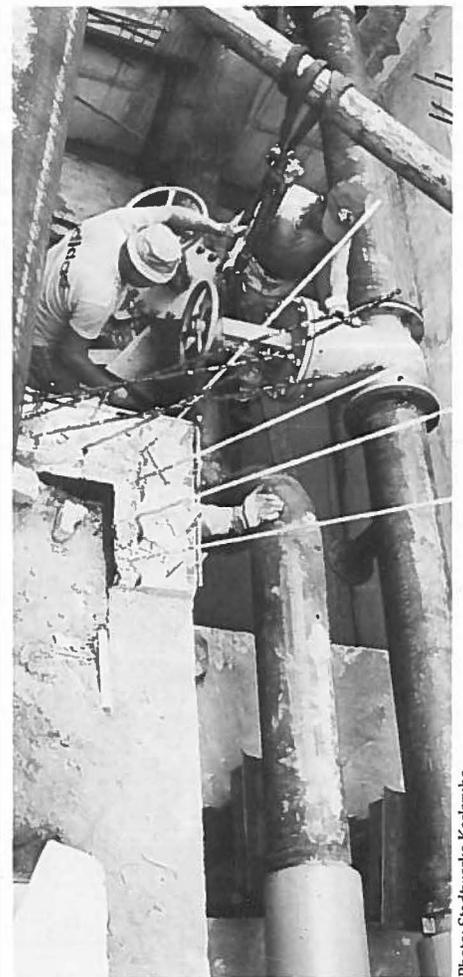
Shut-off valve manhole in Rhode Island Avenue, Karlsruhe. On right, bellows expansion joints to take up longitudinal expansion in the supply and return lines.
