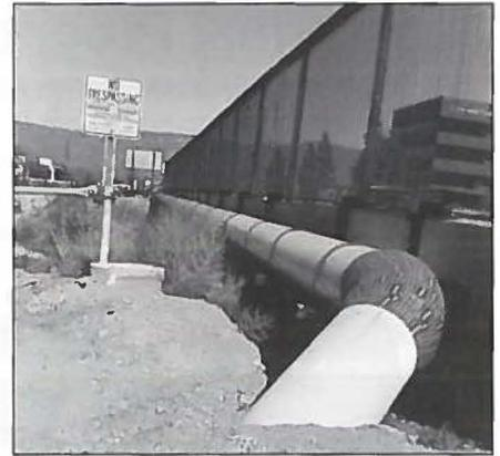
The geothermal transmission main is PVC-covered, pre-insulated ductile iron.
