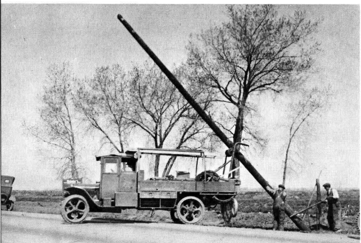
A THREE-MAN LINE CREW sets a line pole using the latest equipment available in the early Twenties.
