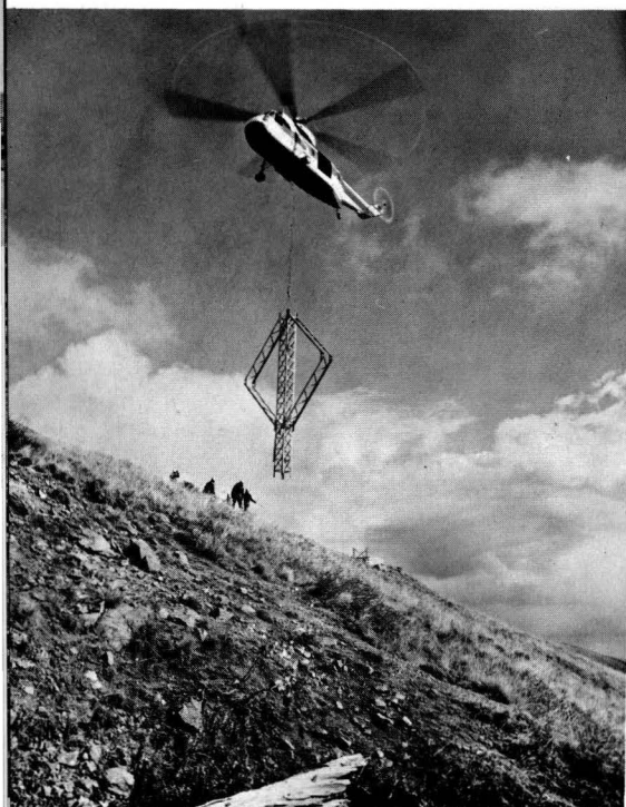
GIANT HELICOPTER is used to set sections of steel towers in place during construction of high voltage electric transmission line between Malta Substation, south of Leadville, and Waterton Substation, southwest of Denver.
