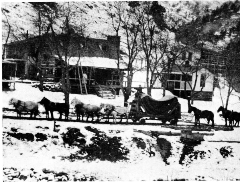
TRANSPORTATION OF EQUIPMENT between Boulder, Colo., and the hydro plant site, five miles up rugged Boulder Canyon, required ingenuity. Here, a 10-horse team inches its way up, pulling a wagon loaded with a section of original generating unit. Horses at rear are a relief team.
