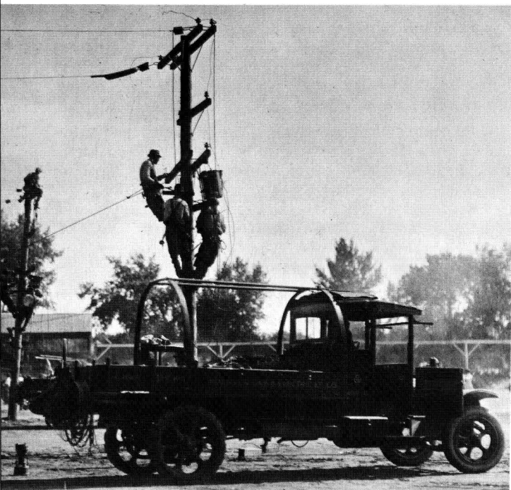
LINEMEN of the Denver Gas and Electric Light Company install a transformer on a distribution line power pole using up-to-date equipment, including a modern line truck of the Twenties.
