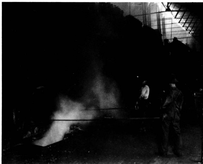
REMOVING THE COKE from the huge retorts in this early day gas manufacturing plant was a hot, tedious and dangerous task. The coke was all that remained of coal which had been baked to release gases that were used to illuminate Denver's first street lights in 1870; and as a fuel for lighting and heating businesses and homes in later years.
