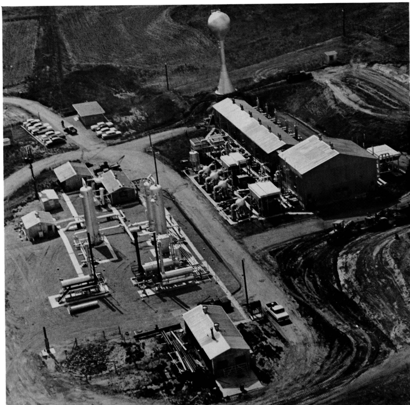
COMPRESSORS AND DEHYDRATING EQUIPMENT are the only evidence of activity at Public Service Company of Colorado's Leyden Mine Gas Storage Project, northwest of Denver. Some 900 feet beneath the ground is the cavern of an abandoned coal mine converted to a natural gas storage reservoir. Operating capacity of the mine is 2.3 billion cubic feet of gas under 250 pounds of pressure per square inch. During periods of intense or prolonged cold, approximately 150 million cubic feet of gas per day can be withdrawn from the mine for use in the Company's distribution system in the Denver area.
