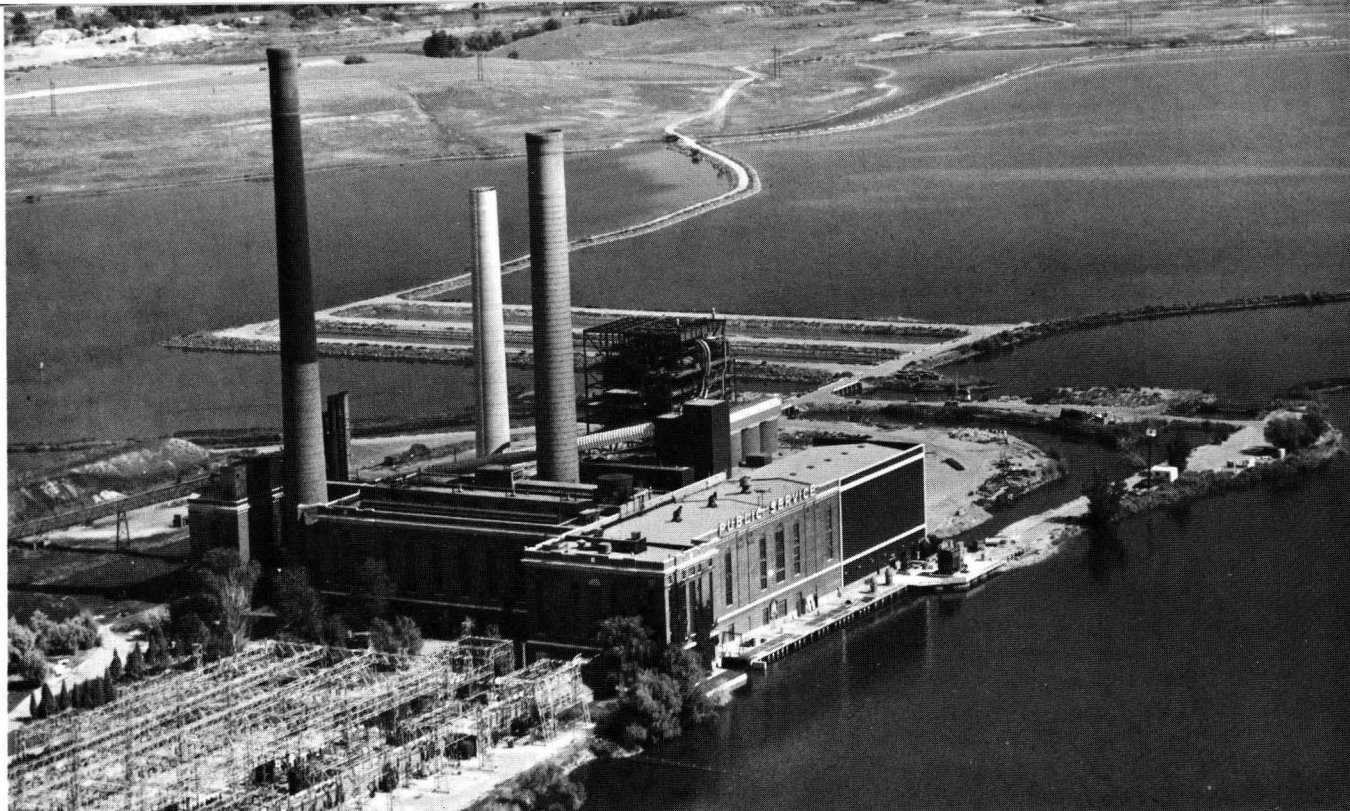
VALMONT steam electric generating station constructed in 1923-24 was the largest powdered fuel generating station between the Missouri River and the Pacific Coast. Present net generating capability of the plant is 300,000 kw.
