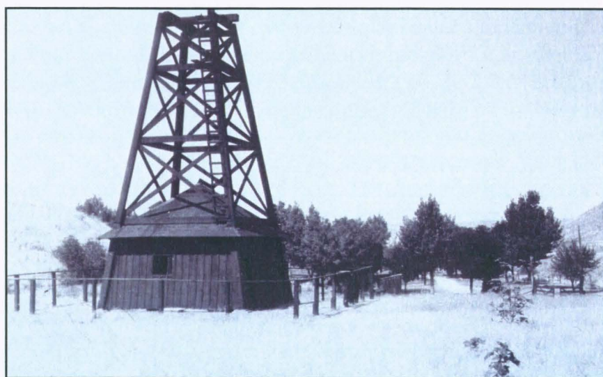
Figure 2. Well House and Drilling Derrick in Hull's Gulch (Circa 1920) 88
