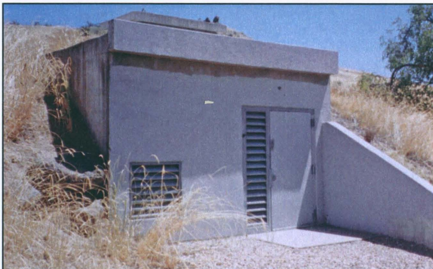
Figure 26. City of Boise Geothermal Well House (photo by author, 2006)
