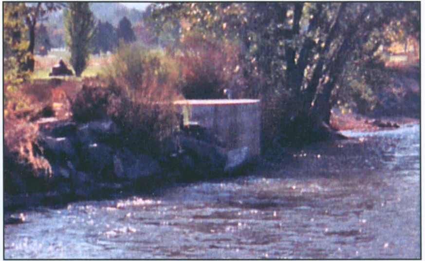
Figure 15. Infiltration Well Constructed near the Boise River in 1952 (Photo by author 2005)
