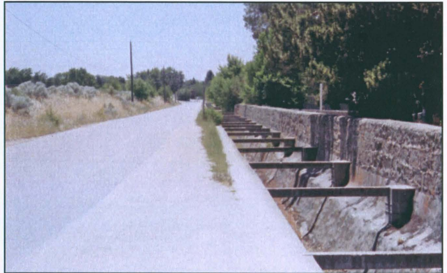
Figure 9. Cottonwood Creek Diversion near Fort Boise (Photo by author, 2006)
