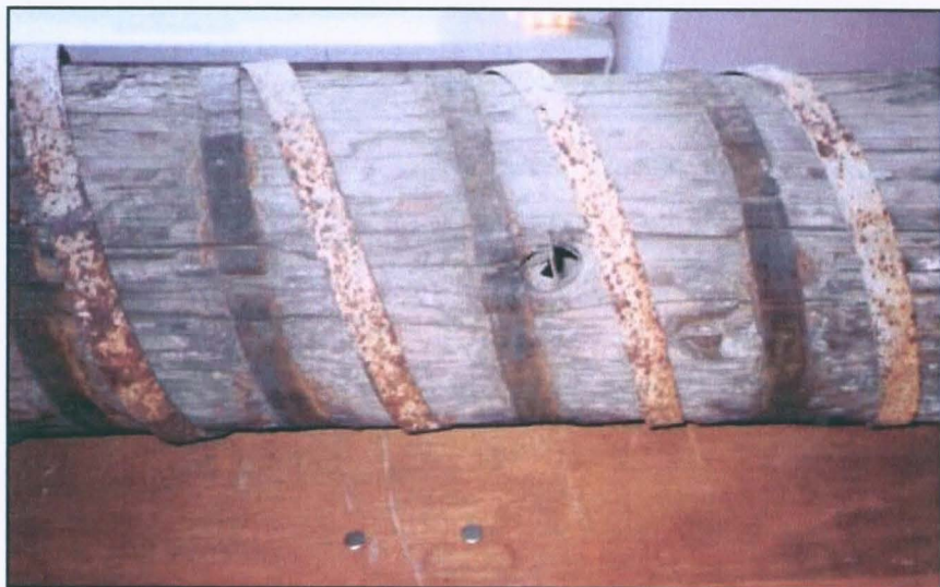
Figure 30. Wooden Water Pipe Used in the Boise Water System. (Photo by author, 2005)
