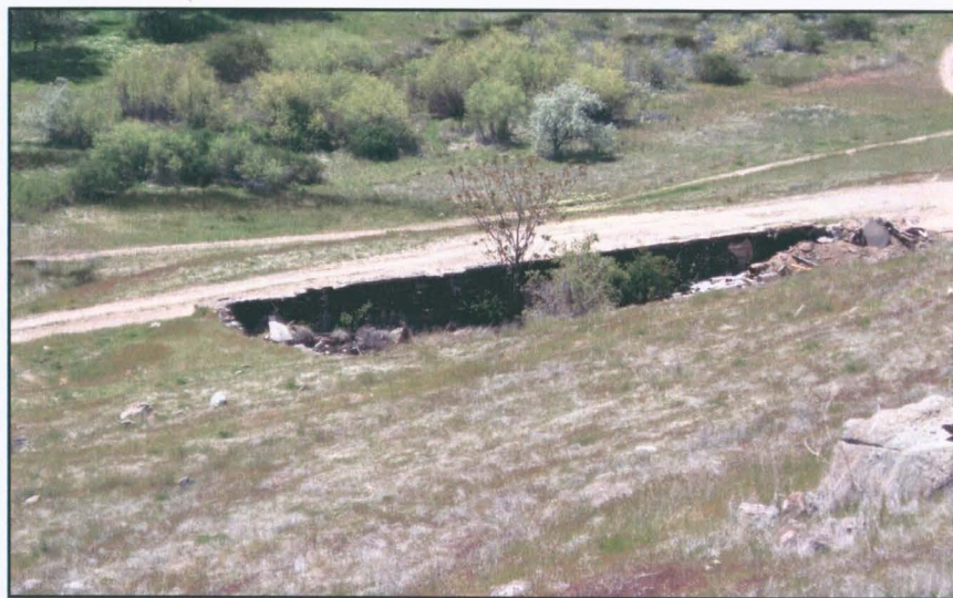
Figure 29. Foundation of Cold Water Reservoir near Hot Water Wells. (Photo by author, 2006)
