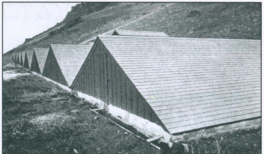
Figure 28. Cold Water Storage Reservoir near Hot Water Wells (circa 1920) 189
