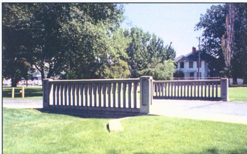
Figure 8. Guardrails of Bridge Over Walling/Perrault Canal near Old Fort Boise (Photo by author, 2006)
