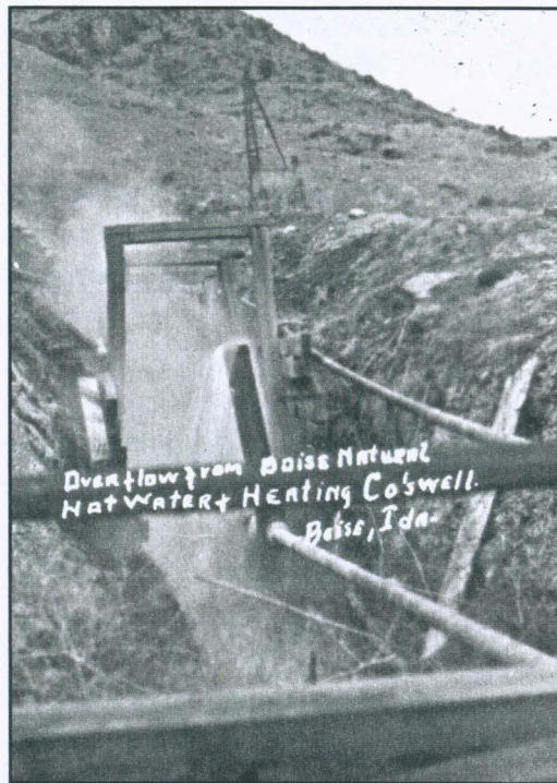
Figure 24. Hot Water Overflow from Geothermal Well 171
