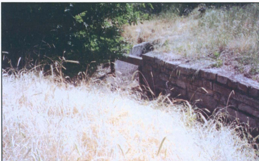
Figure 7. Remnants of Perrault Ditch at Warm Springs Avenue (photo by author, 2006)
