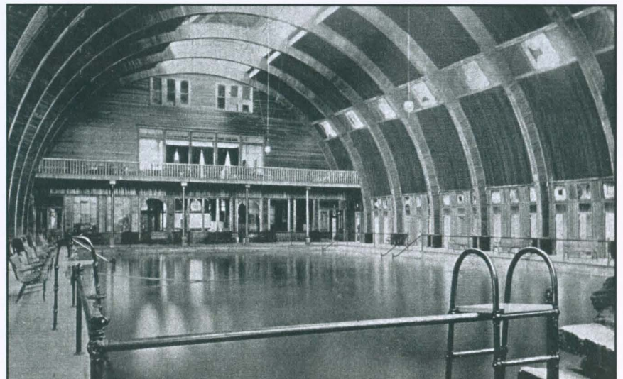
Figure 27. Natatorium Plunge Pool and Roof Support Arches 185
