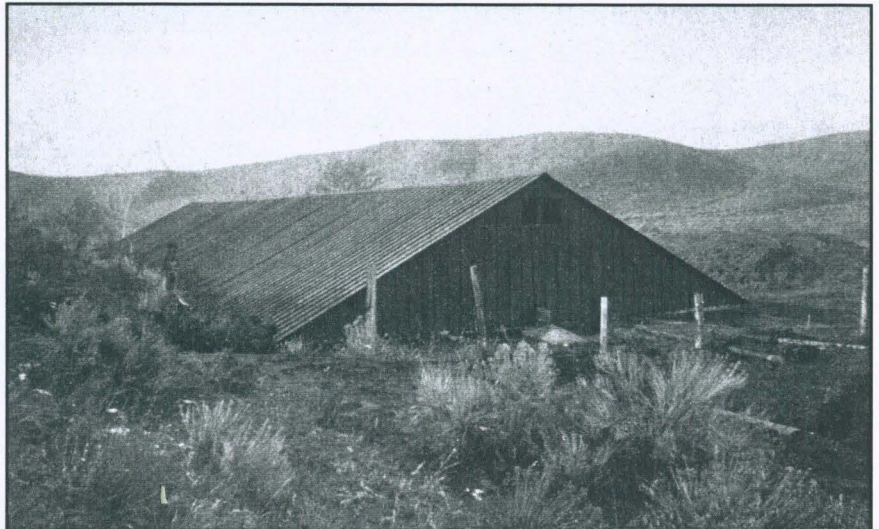
Figure 12. Water Reservoir No. 2, Hull's Gulch 122
