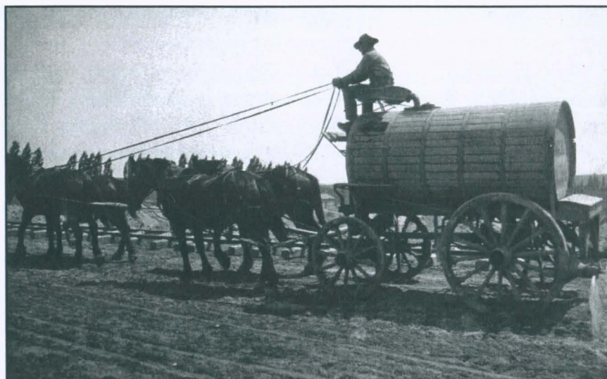
Figure 34. Water Sprinkler Wagon, Deer Flats Reservoir. 264
