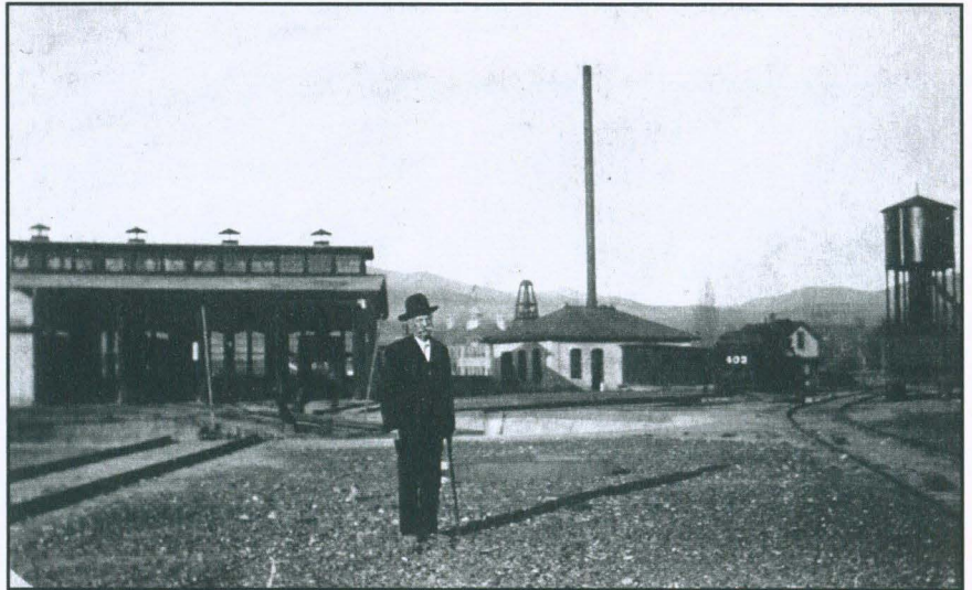
Figure 19. Oregon Short Line Railroad Water Storage Tank 155
