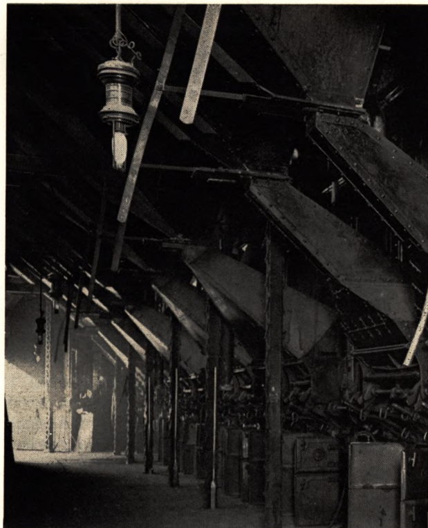
Arc lights of the kind shown here, above the aisle in Kentucky Avenue boiler room, were used in older plants.
