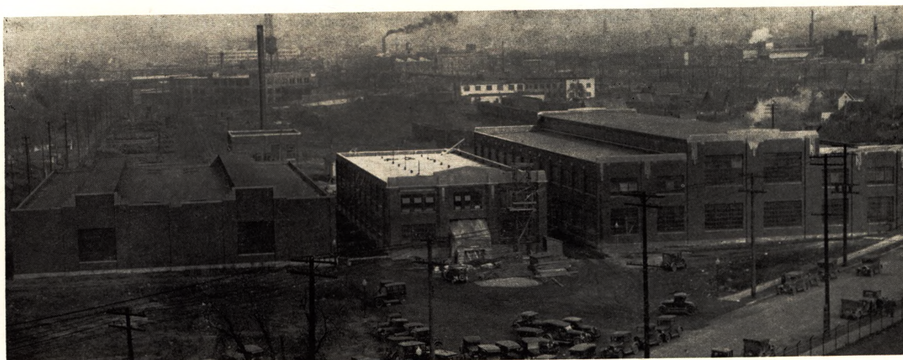
Construction of this operating and engineering center in 1927, at 1230 West Morris st., was a major milestone in the development of electric service for Indianapolis.
