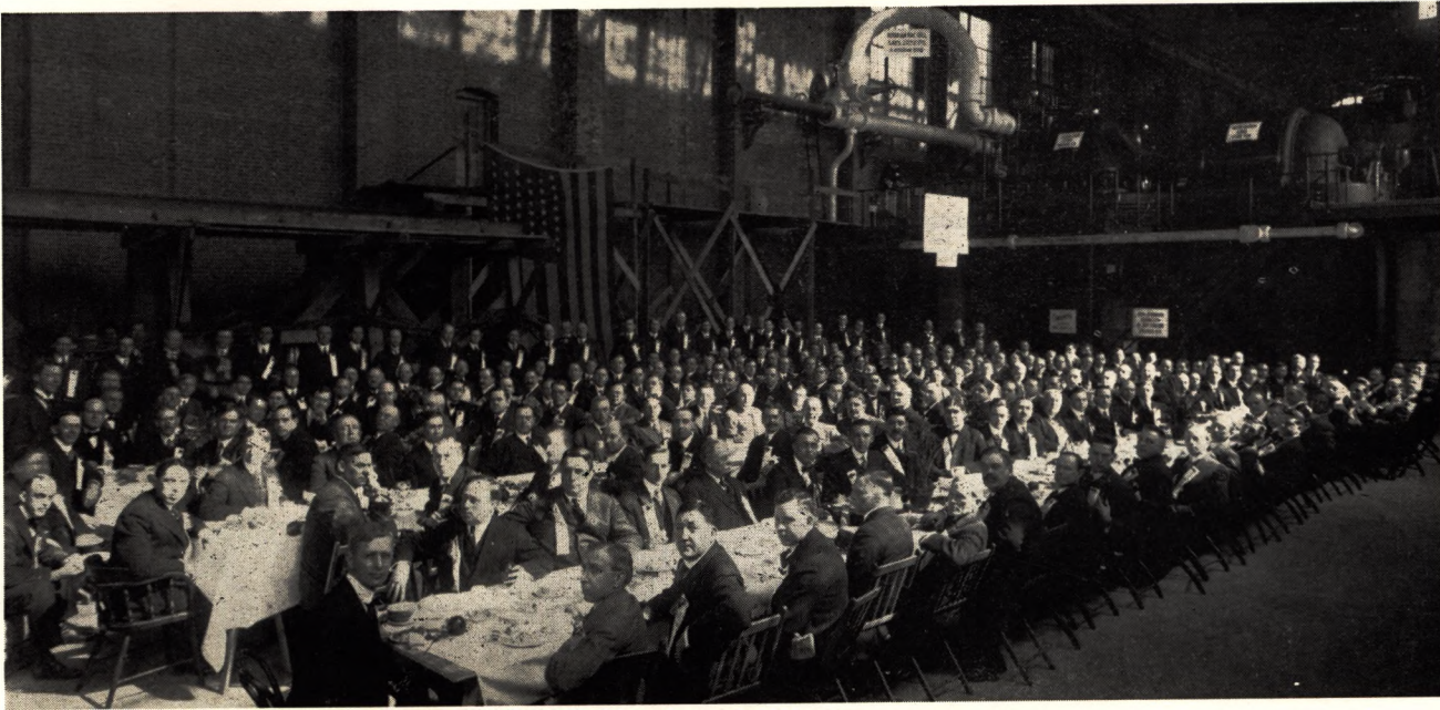
The Rotary Club met in Mill Street plant Jan. 15, 1915, to see the 10,000-kilowatt turbo-generator shown at rear, which had just been installed by Indianapolis Light and Heat Company and was called "the largest and most economical power and light producer in the state of Indiana." This machine was wrecked by explosion April 2, 1923.
