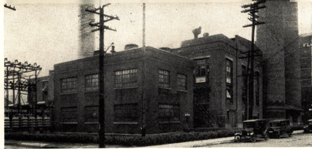
West plant of Merchants Heat & Light Company at 744 Washington ave., built originally in 1909-10.
