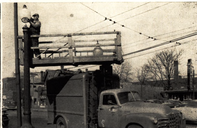
Cleaning street lights in 1919 was a job for three men, a boy and a horse and wagon, as it appears in the picture at left; and in 1954 it is done with special trucks of type shown at right, with one man working on the high platform and another man washing globes inside the truck.
