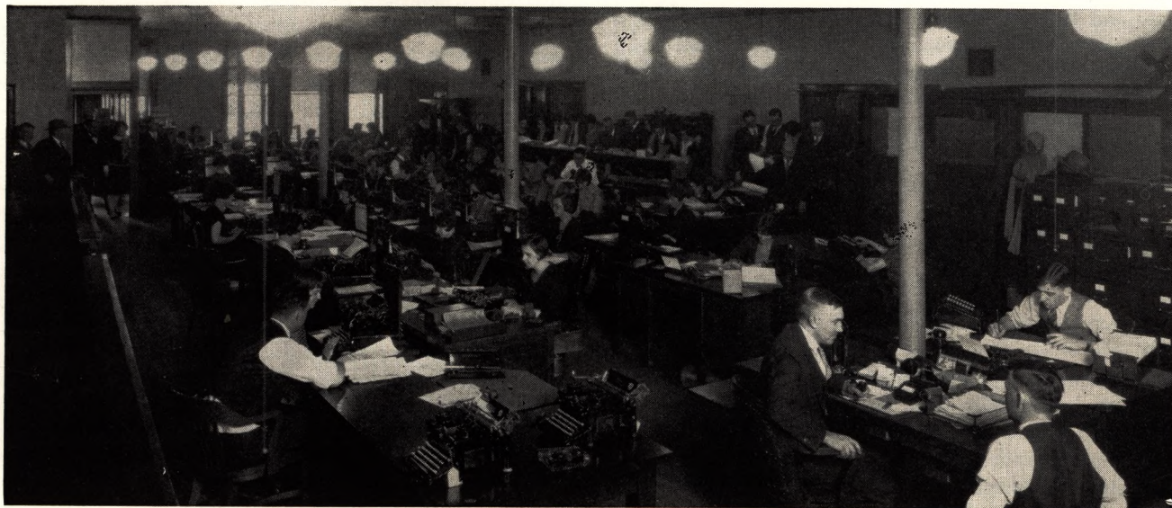
General accounting office of Indianapolis Light and Heat Company, on fourth floor of 46-48 Monument Circle building in November, 1926, when preparations were being made for merger with Merchants Heat & Light Company to form the present Indianapolis Power & Light Company.
