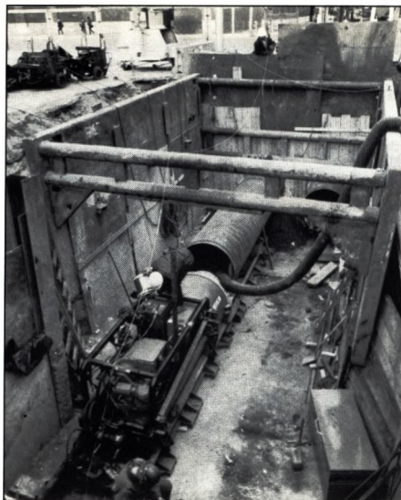
Construction of the piping distribution system in the downtown area was successfully completed and the streets restored prior to the start of the NCAA Final Four Basketball Tournament.
