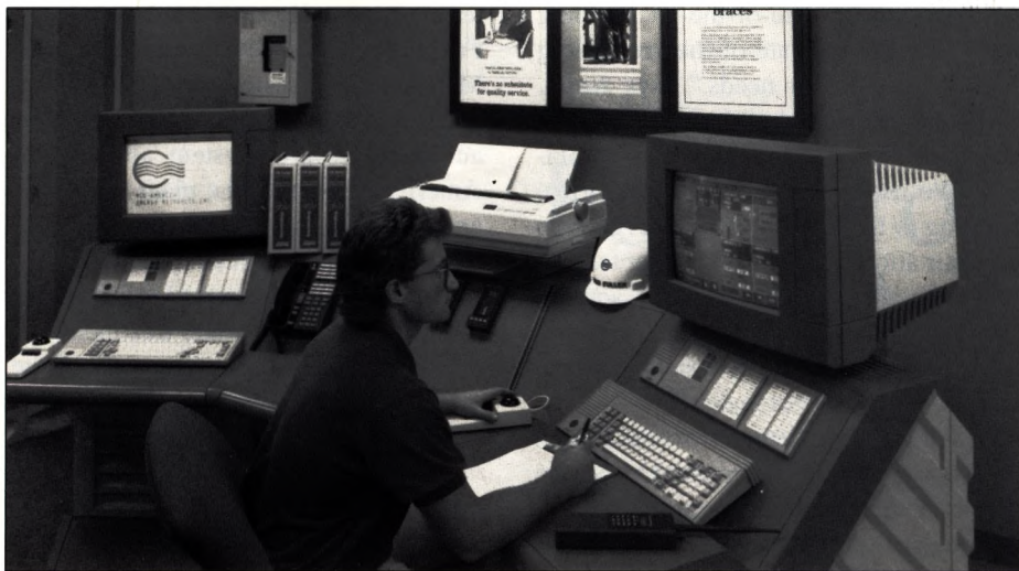
Mid-America's state-of-the-art computerized control and metering systems help keep the system running smoothly.
