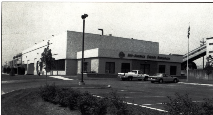
Mid-America's new district cooling plant began construction in summer 1990 and was ready to supply chilled water in spring 1991.
