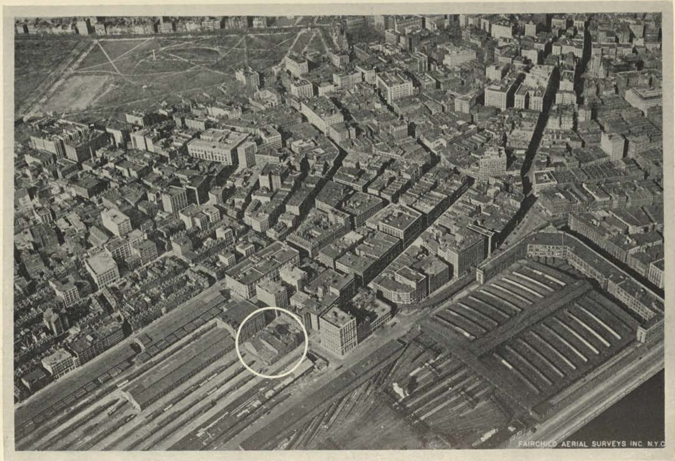
The uptown section. Location of Station S-2 is shown in white circle
