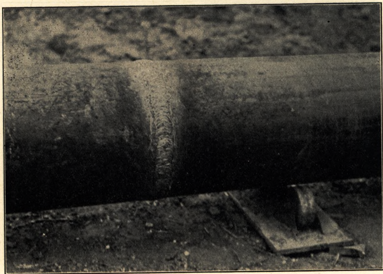
FIG. 1—Typical butt weld.
