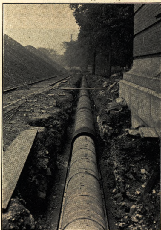
FIG. 4—Pipe insulated and waterproofed. Sheet metal conduit partially placed.
