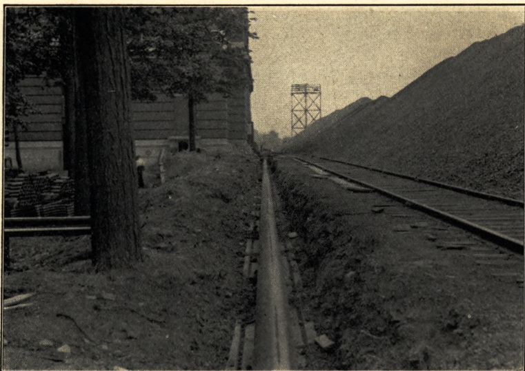
FIG. 3—Pipe aligned and welded ready for covering.
