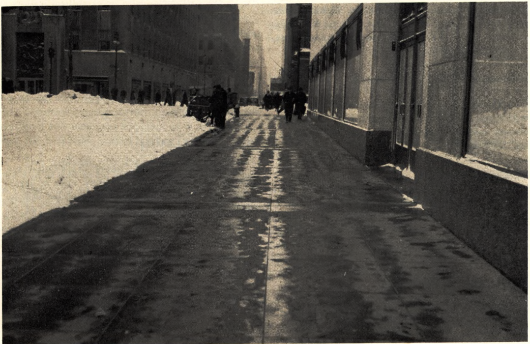
The excellent job of snow melting being done by the sidewalk installation in front of Best & Company's new store on Fifth Avenue, New York City, is indicated by this picture.
