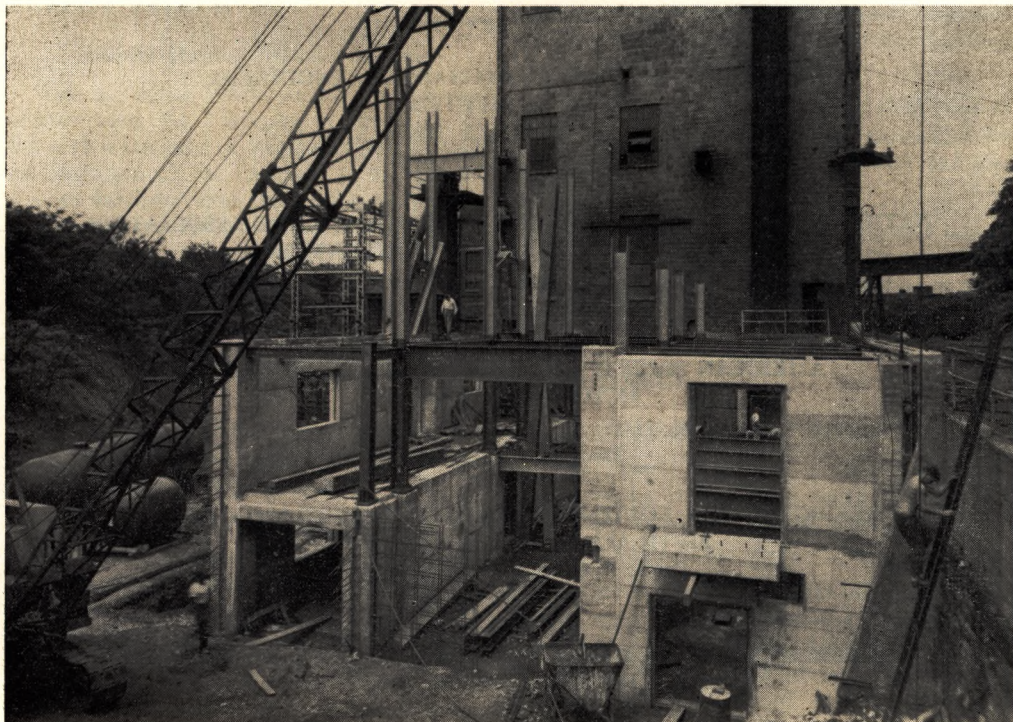
Beech Street Heating Plant Addition, Akron Ohio.
