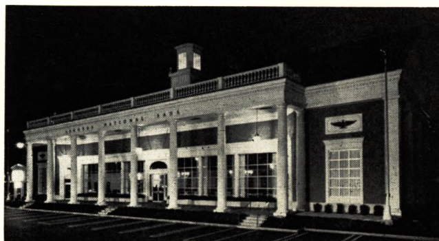
New buildings like the Lagonda National Bank in Springfield, rely on Ohio Edison steam for space heating. And others, like the Youngstown University buildings, are also cooled in summer by steam.
