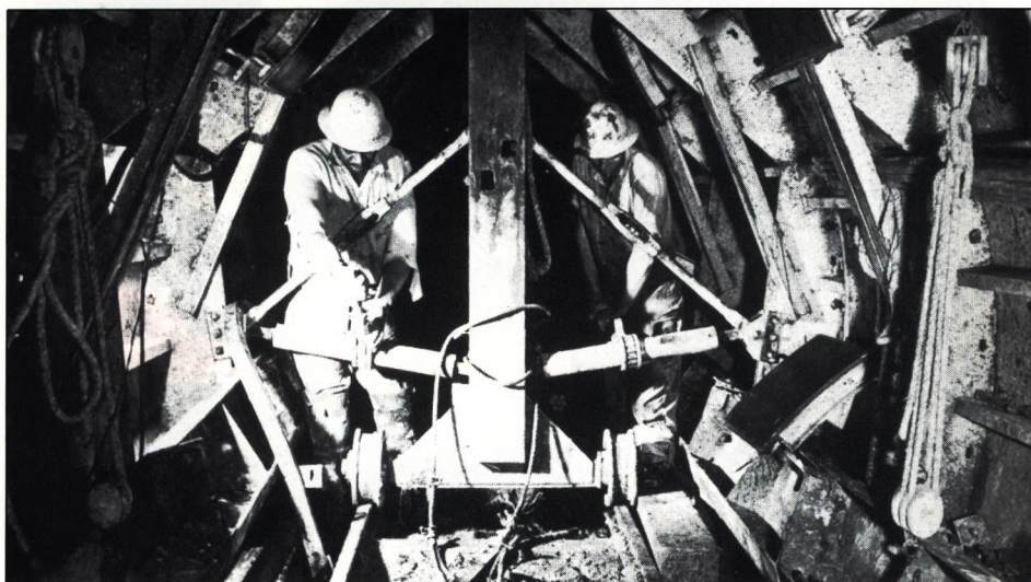
1950 Construction phase of the tunnel 50' below the Schuylkill plant to West Philadelphia.
