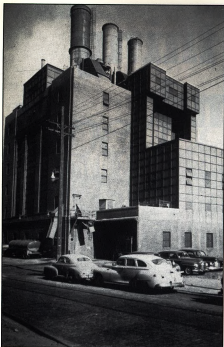
The Willow Station, shown here in the 1940's was Philadelphia's first plant dedicated to the production of district steam.
