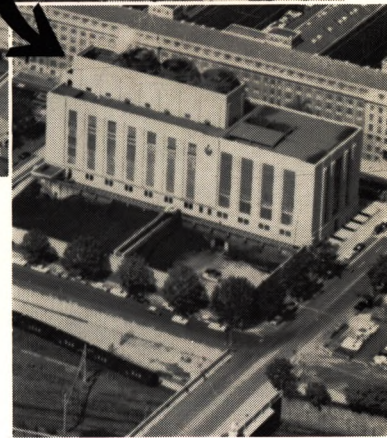
Central Heating Plant Washington, D. C.
