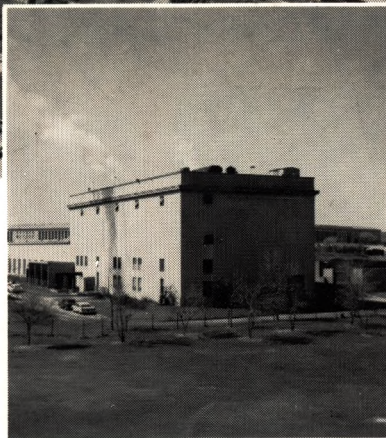
Arlington Heating Plant Arlington, Virginia
