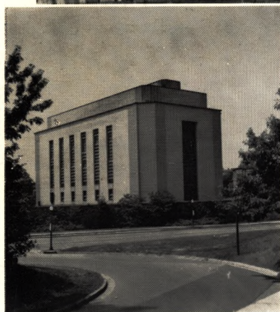
West Heating Plant Washington, D. C.
