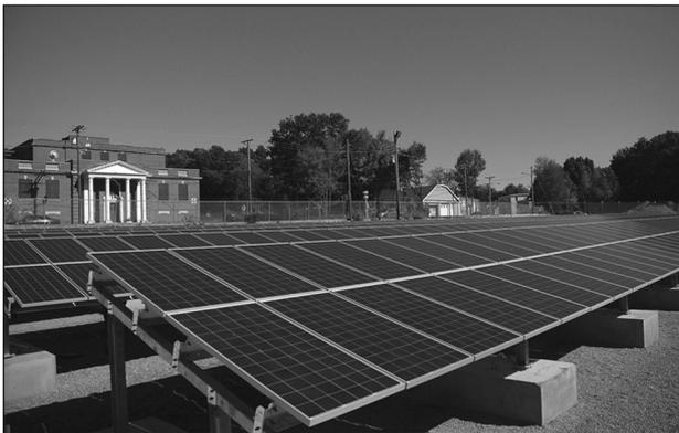
**Solar Panels, located adjacent to the New Water Treatment Facility, provide 10-15% of the plant's energy needs.**
