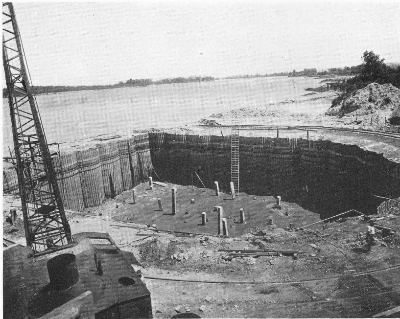
Plate IV: Cofferdam immediately after being unwatered.
