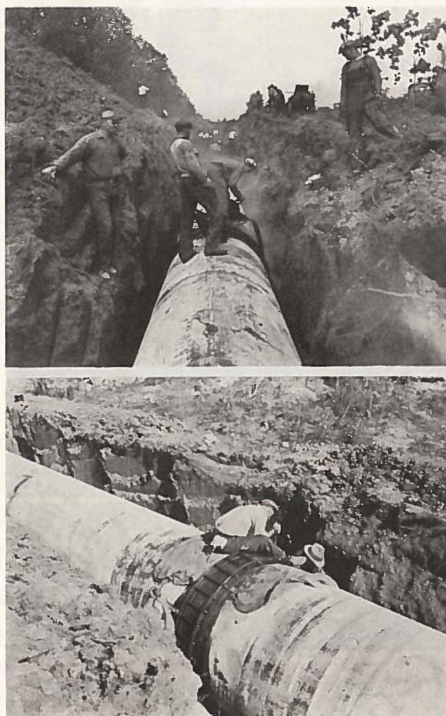
Upper—Applying Field Enamel Coat on Coupled Joint. Lower—Tightening Bolts in Dresser Couplings.
