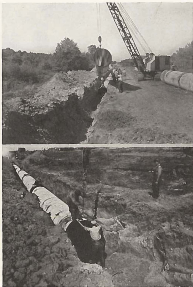
Upper—Lowering Pipe Into Trench. Lower—Installing Coupling Middle Ring on End of Pipe Section Already Laid.
