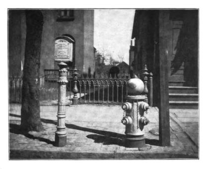
FIG. 1. - HYDRANT AND CALL BOX FOR FIRE BOAT PIPE LINE.
