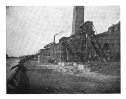
FIG. 2. — ICE ELEVATORS AT SHORE SHAFT.
