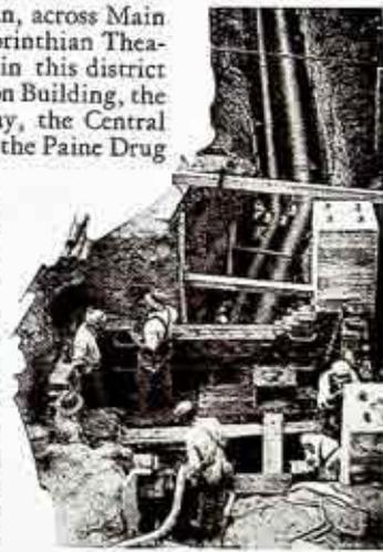
Steam manhole in line serving the General Railway Signal and Symington Companies in process of construction. It is located just across the N. Y. C. tracks, at the south end of Station Nine's steam bridge.
