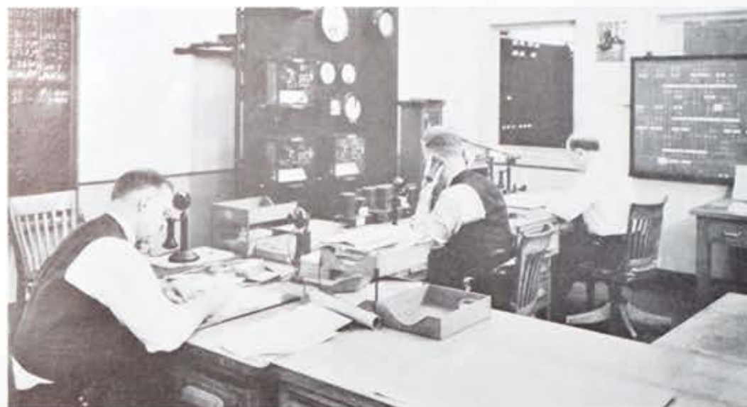
Scene in the power load dispatcher's office at Station Three. From left to right are shown chief load dispatcher S. S. Summers, and dispatchers Harold McDonald and George Love. In this office continuous calculations are made for the disposition of the load between stations. The load dispatcher predicts tomorrow's load requirements today and makes necessary plans for procuring the necessary generating capacity, apportioning the load between steam, hydraulic and Niagara power as circumstances of weather and demand indicate.
