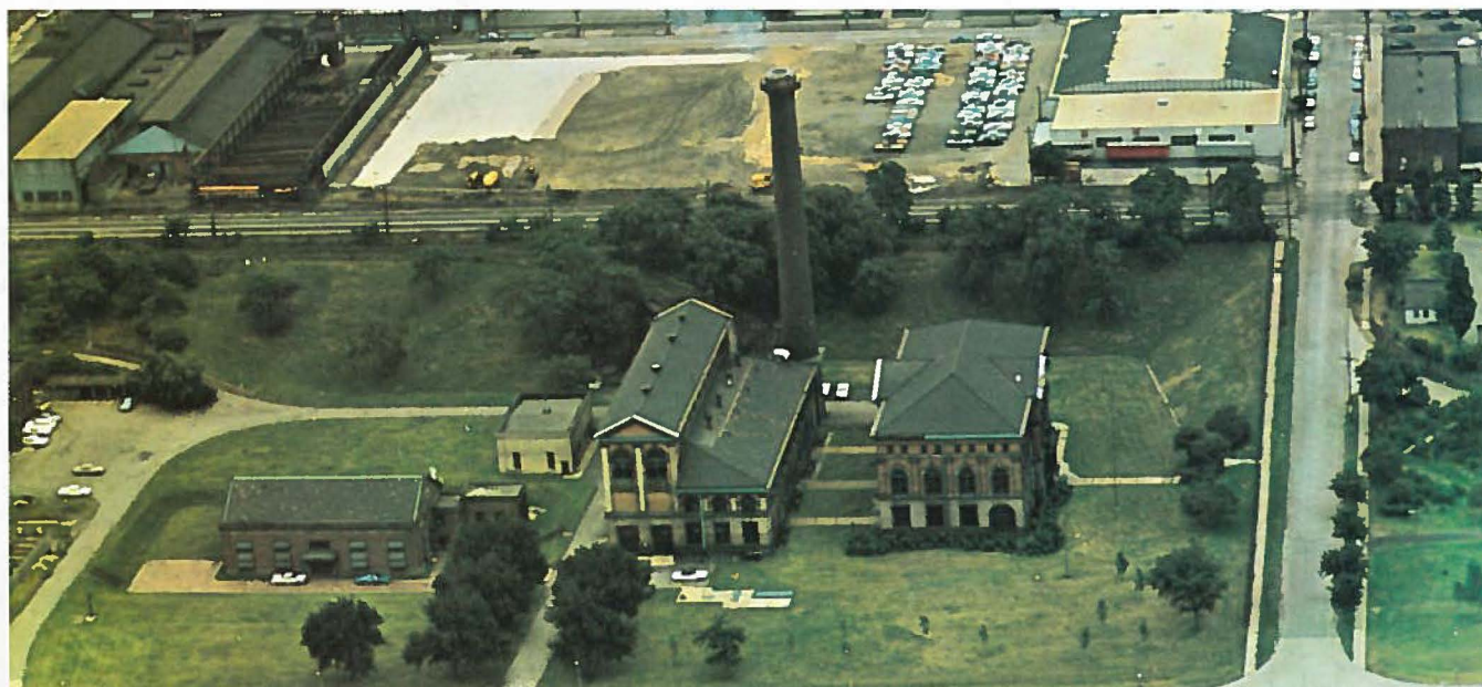
Kirtland Raw Water Station, in service since 1904, is scheduled for replacement by a $5.3 million all-electric facility. Present steam pumps at the lakefront plant draw water through Crib No. 3 and move it to Fairmount Reservoir.
