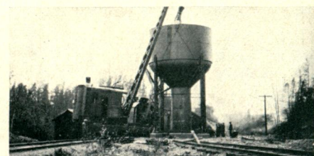
Placing tank on new foundations four miles from former location.
