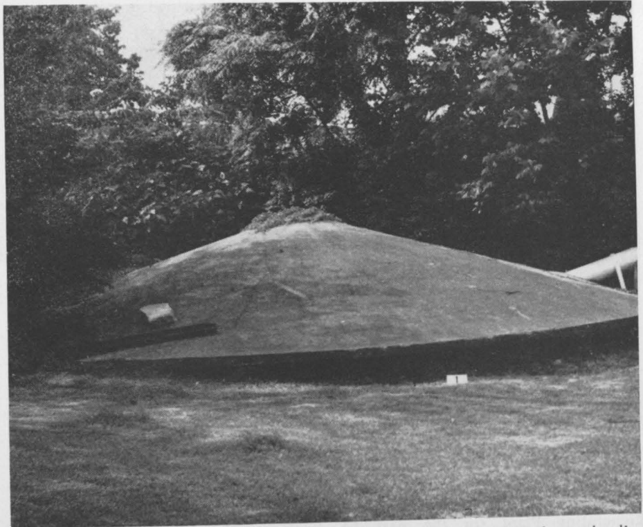
ORIGINAL PUMPING RESERVOIR for Houston Water Works in 1879, located adjacent to Bayou Pumping Station near downtown, is in use in present system.
