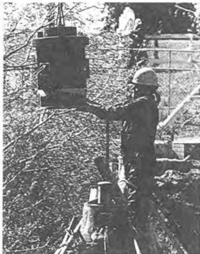
Pump mechanic John Tracy Lyon installs a new motor at the Rolling Hills #1 pump Los Osos. Though not visible, the motor is being dropped into place by a helicopter due to the inaccessibility of the location of the pump.
