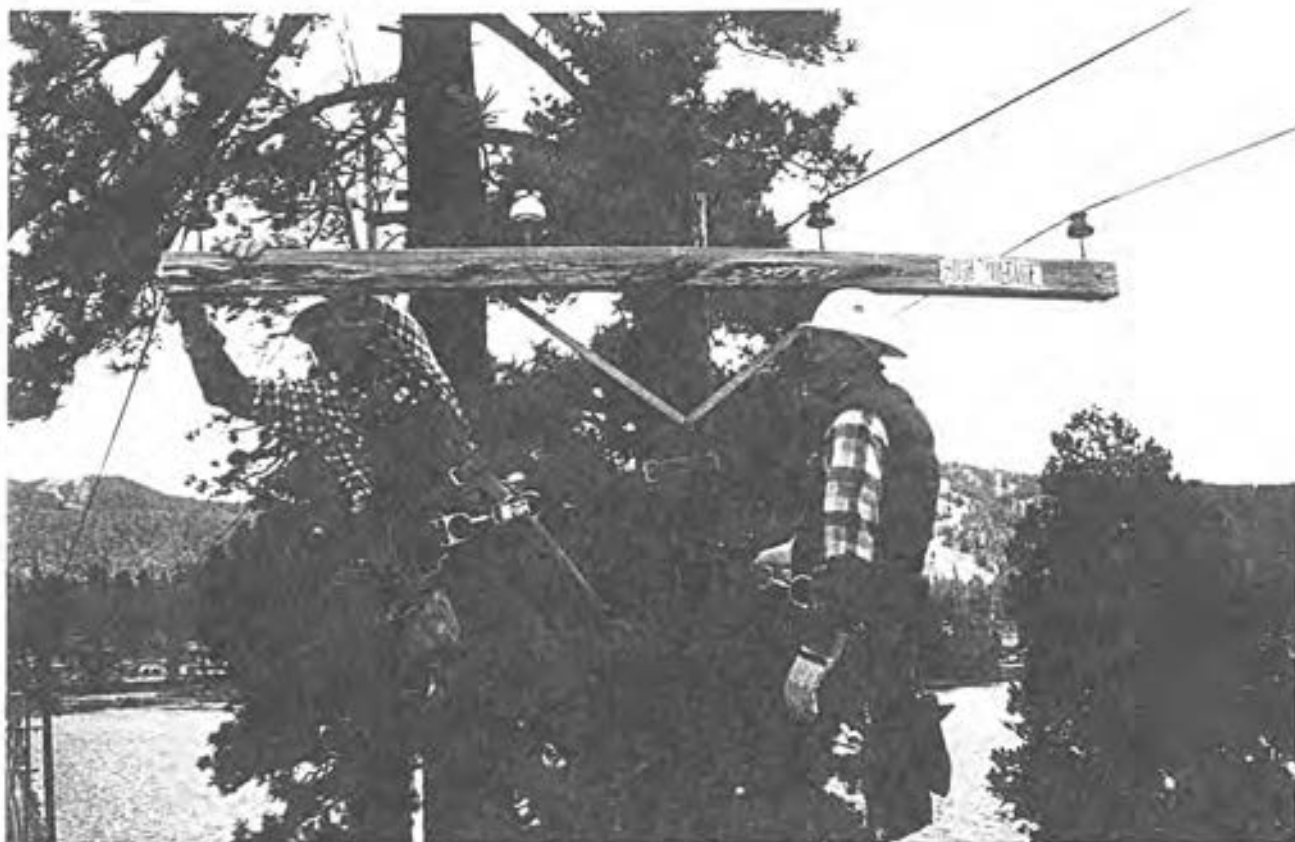
SCWC's Bear Valley Electric lineman David Burks and Service Crew Foreman Bob Bacon tighten hardware on 4KV circuit, high above Big Bear Lake.
