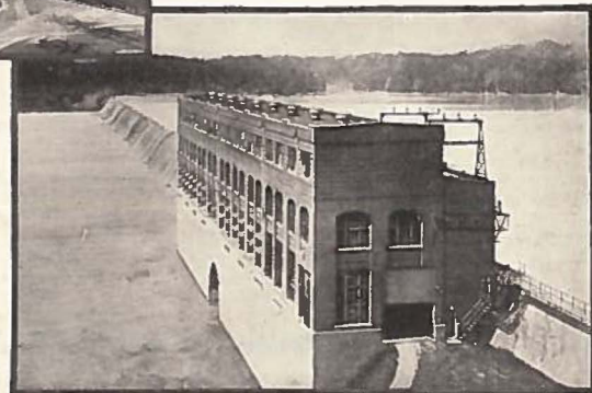
Hydro-electric station of Broad River Power Company at Parr Shoals, South Carolina. Capacity 14,880 kw.
