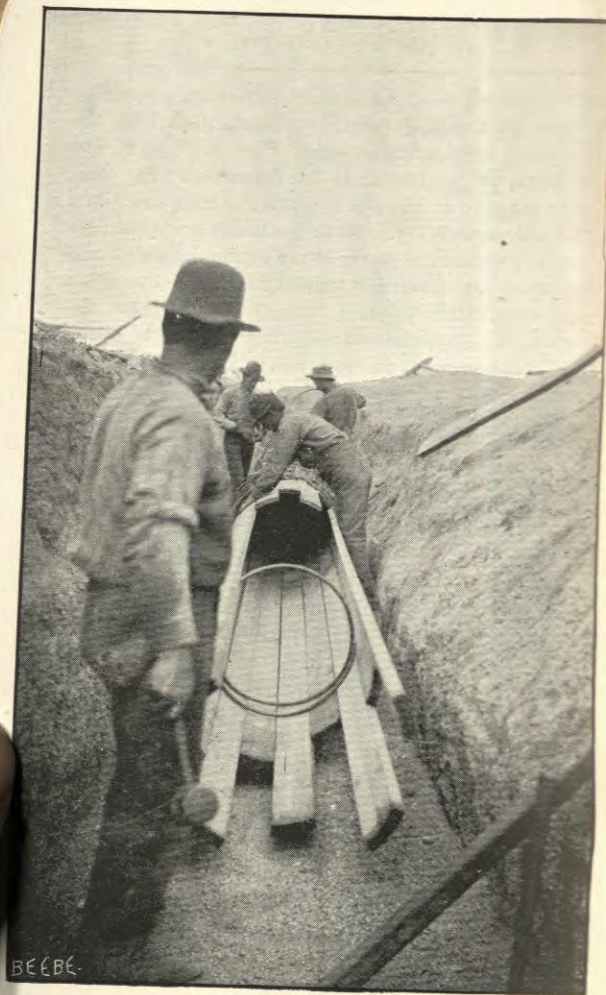
ERECTION OF PIPE.
