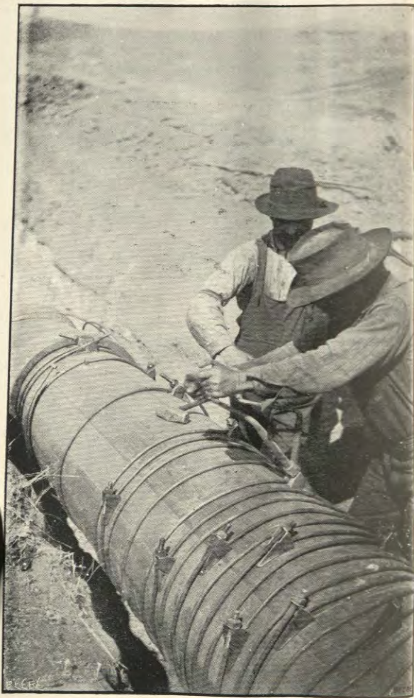
WOODEN PIPE REDUCING FROM 24 TO 20 INCHES TO CONNECT WITH 20-INCH IRON PIPE.
