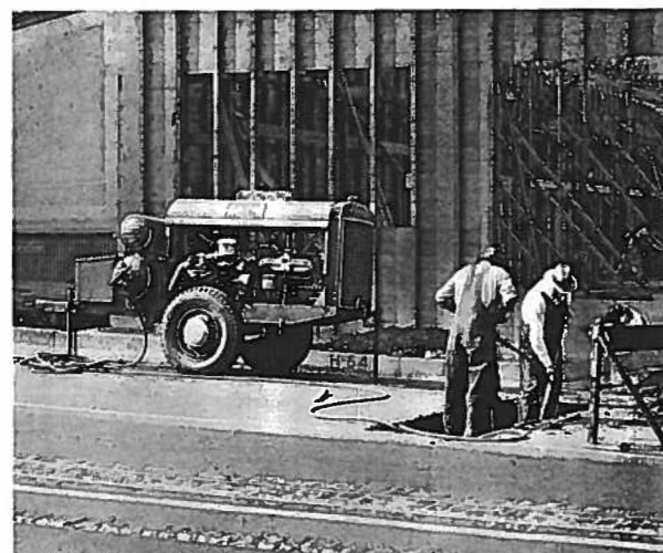
Fast-towing Worthington portable air compressor, driving Worthington pavement breaker and clay spade, serving a western city.
