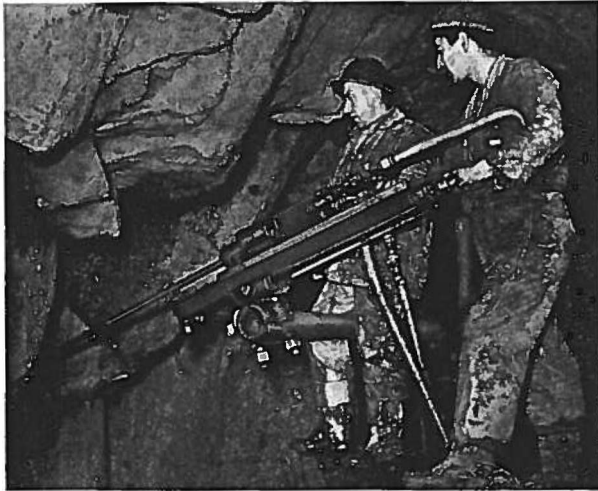
Worthington pneumatic-feed drifter drill, at the San Jacinto Tunnel, Metropolitan Water District of Southern California.
