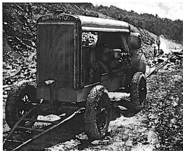
Four-wheel Worthington portable air compressor operating rock drills on large highway construction job in the South.
