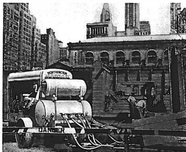
Worthington portable air compressor on construction of Sixth Avenue Subway, New York City.
